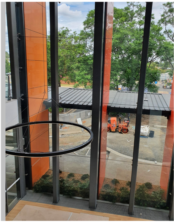
The view of the double-storey glass front entry from the first floor of the new Macquarie Building.
